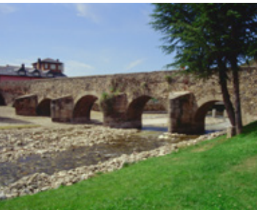
Medieval bridge in Molinaseca
