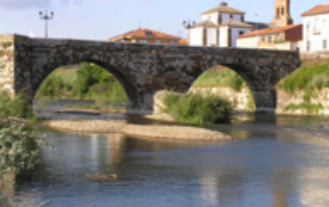
Bridge over the River Orbigo
